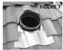
to double seal any potential water leaks. Finish installation by following STEPS 2 and 3 of Shingle Roof instructions.
