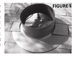
**STEP 2:** Once the flashing has been secured to the roof, mount louver ring onto flashing (**Figure 2**), and secure with (4) #8 x ½" self-tapping stainless steel screws (*supplied*; **Figure 3**).
