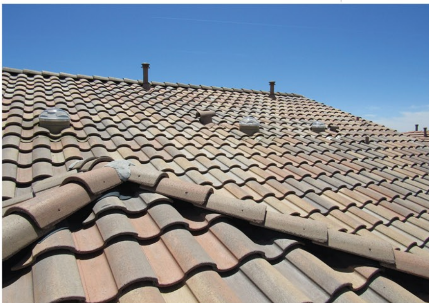
Tubular skylights easily install on s-tile roofs. Photo courtesy Elite Solar Systems
