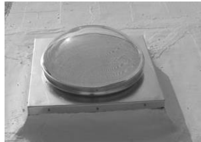
** Examples of installed Curb Flashing.
